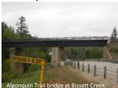
Algonquin Trail bridge at Bissett Creek
